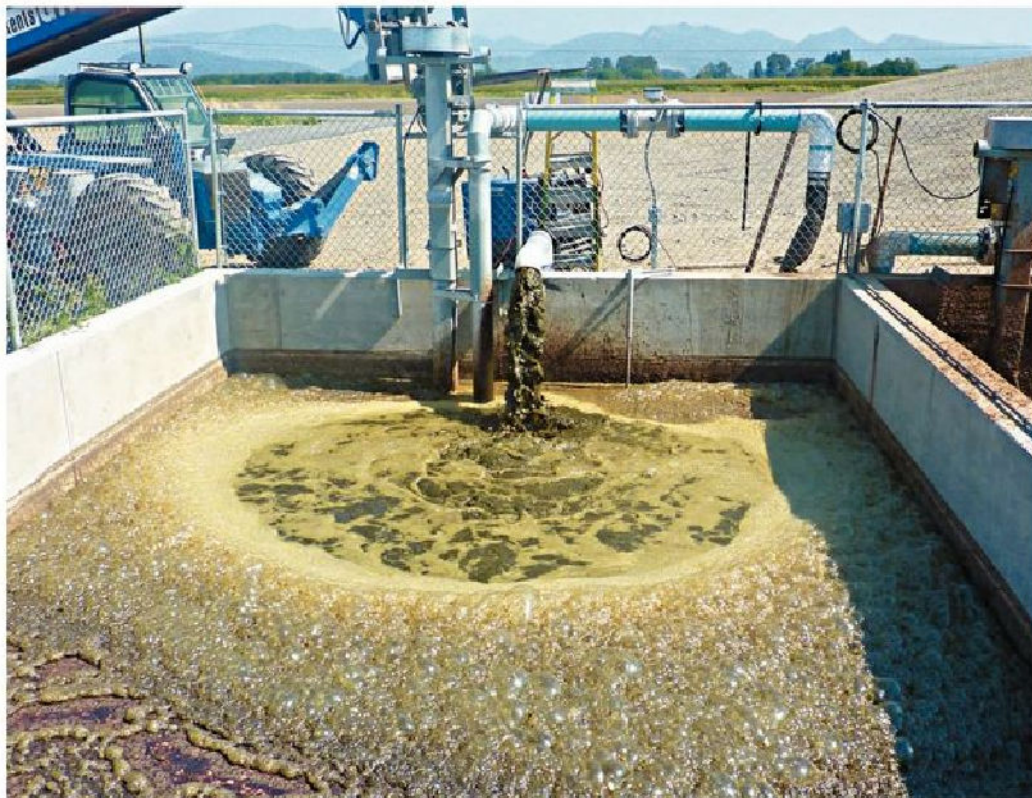
'BEAUTIFUL STUFF': Liquids from the end of the digester process are poured back into the holding tank and will later be used on fields
